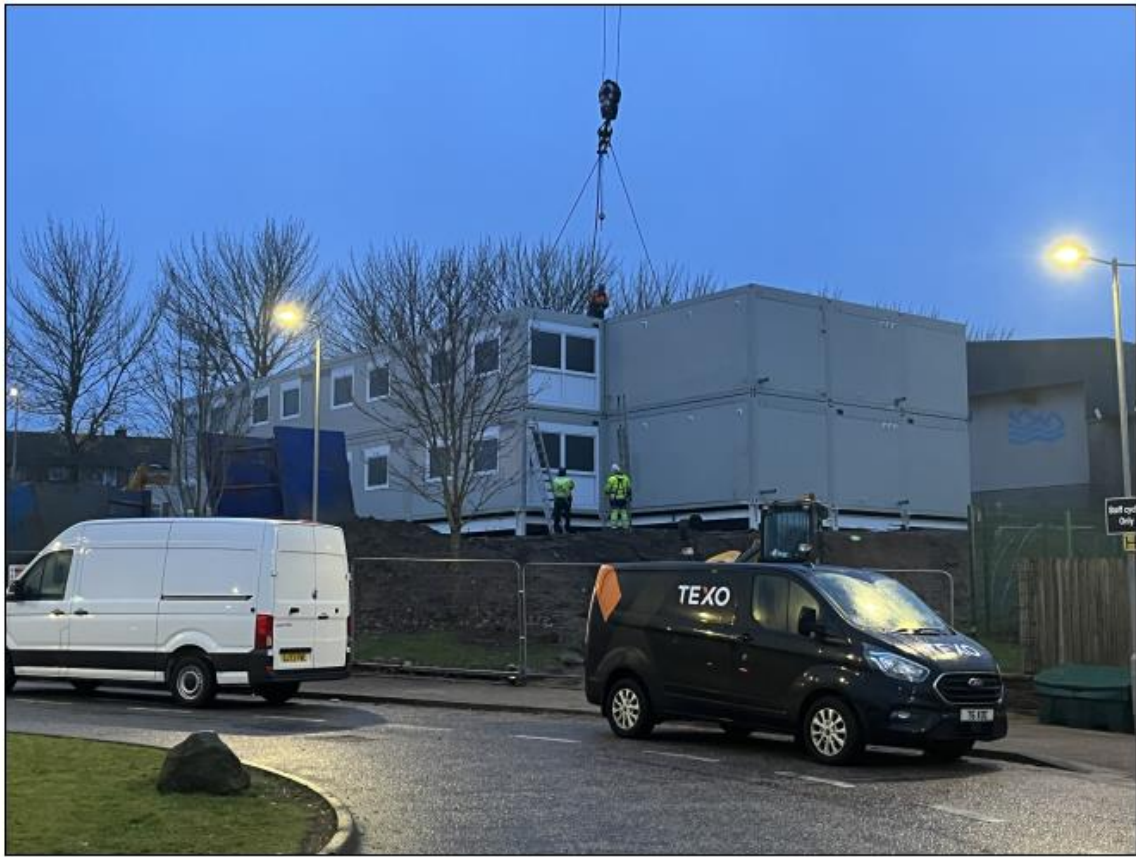
Installation of the units
