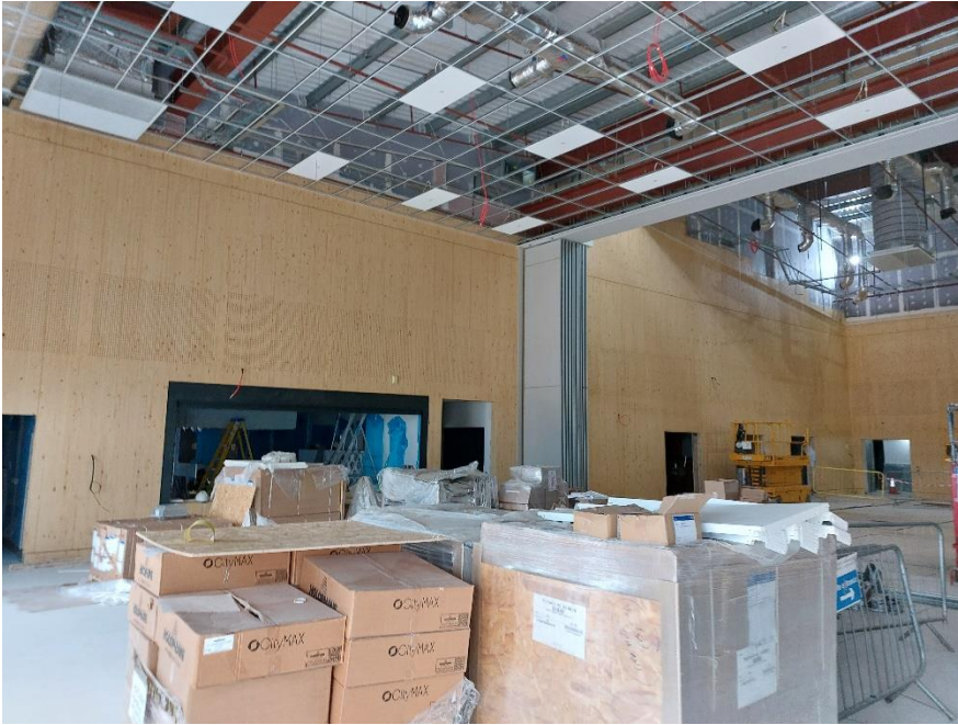
Dining and Assembly Hall progress
